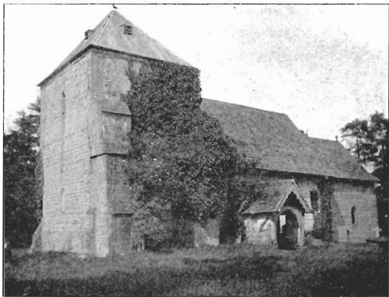
CHURCH OF ST. MARY (BEFORE REPAIRS).
