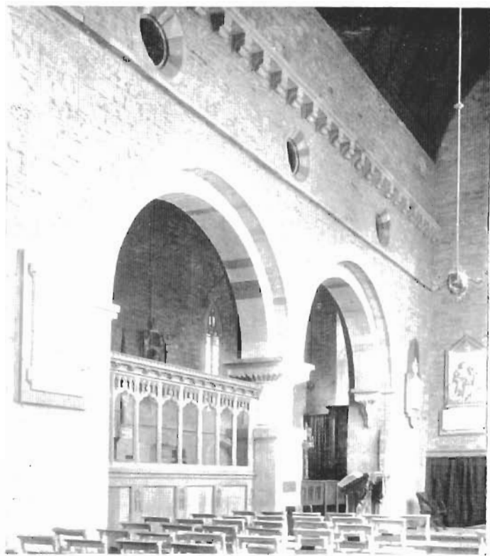
SOUTH AISLE, showing Corbel-table of Norman roof and dripstone under Clerestory Windows.
