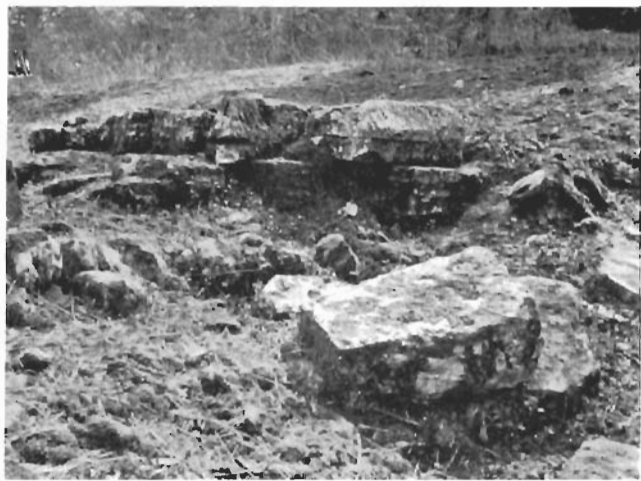
Fig. 3. Southwest angle above quarry—fallen block
