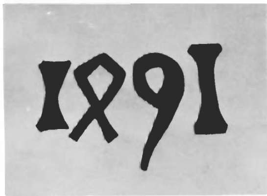
DATES CUT ON SOUTH WALL, CHEDWORTH CHURCH
