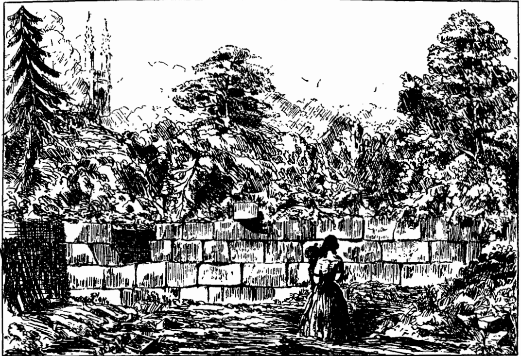
SECTION OF THE CITY WALL EXPOSED FROM BRUTON LANE
