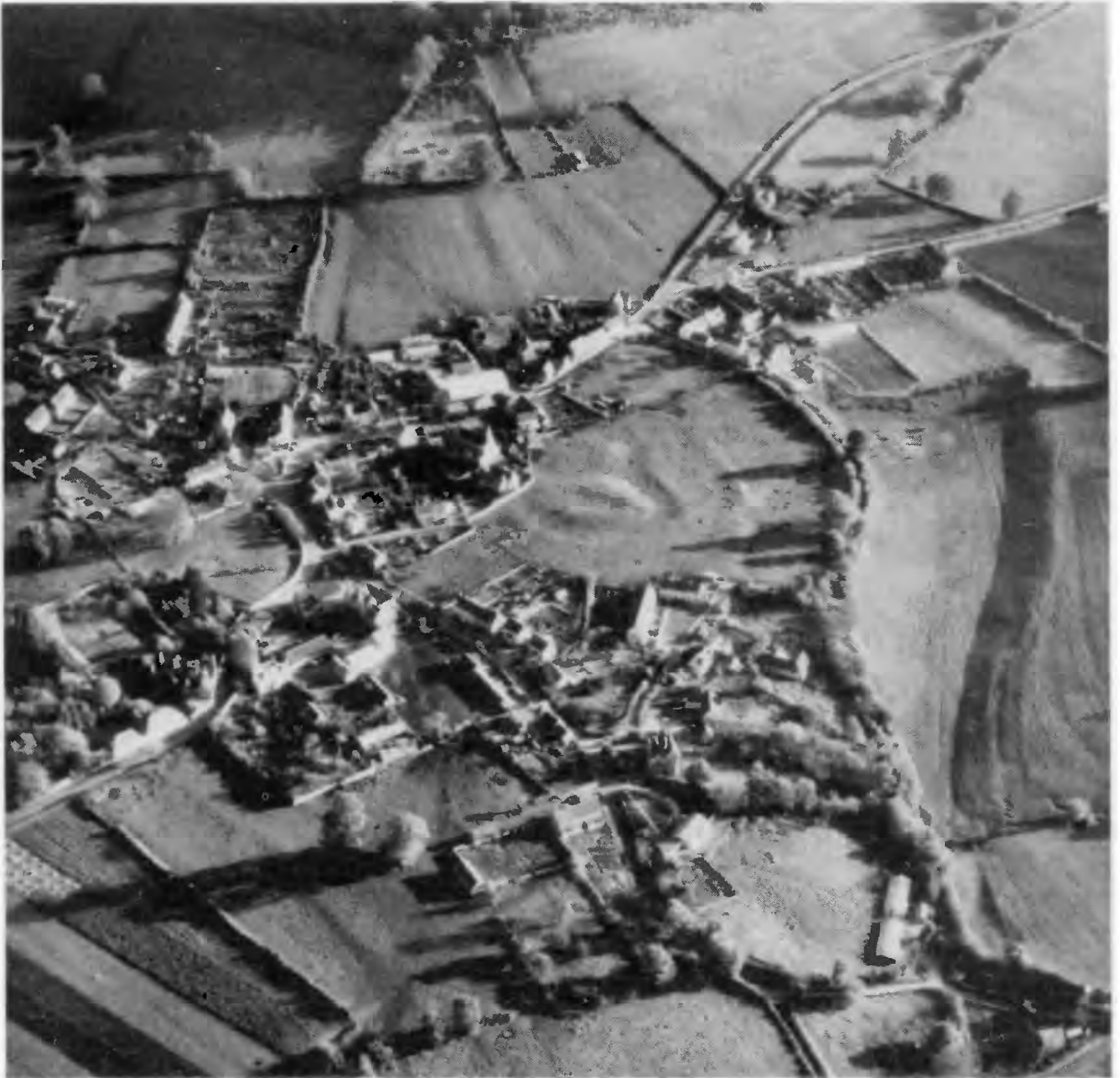
FIG. 2 Aerial view of Hillesley taken November 1965 from the north-west. The earthworks on Very Croft are visible in the centre of the picture. (Photo: Cambridge University Collection, copyright reserved.)
